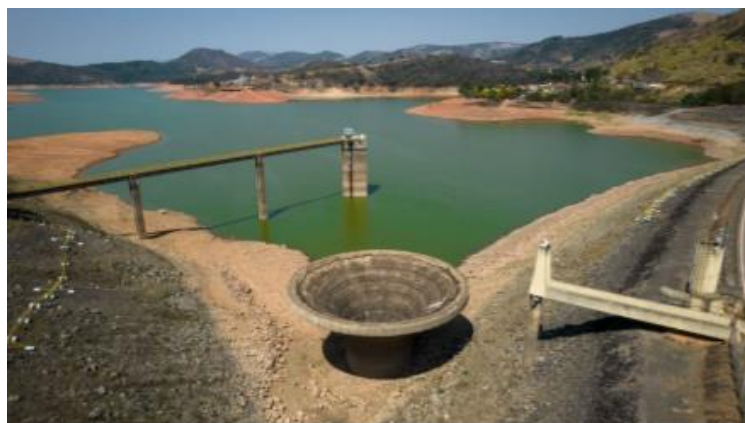
Brazil relies on hydroelectricity for more than 60% of its power, and the drought has forced the country to increase output of more expensive and carbon-intensive electricity. [Photographer: Jonne Roriz/Bloomberg]
